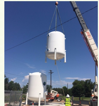
Installation of GAC Filter Unit at Aga Park.
